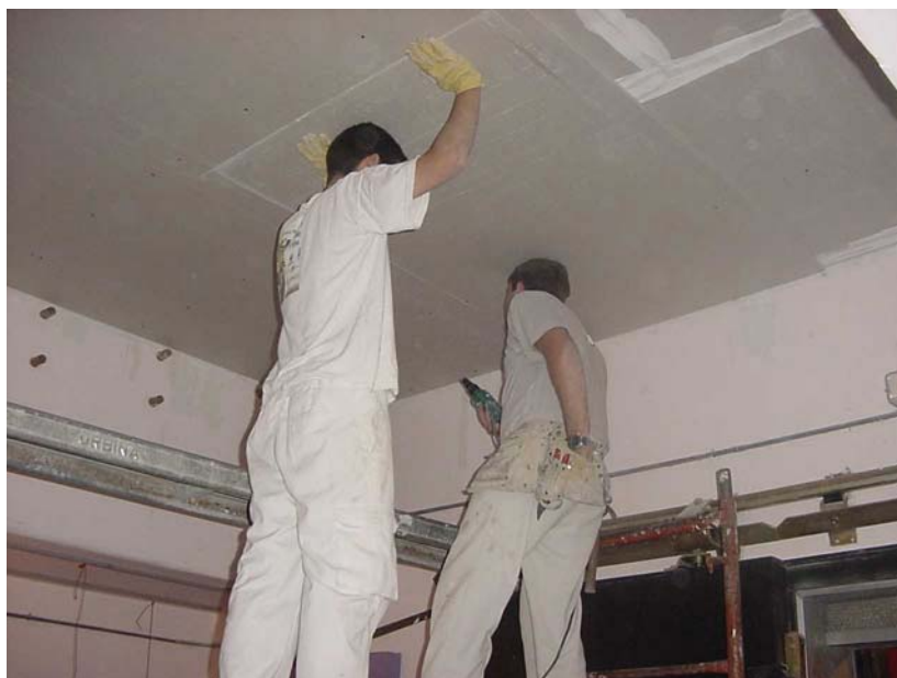
Photo 4: Mounting of the second plasterboard
