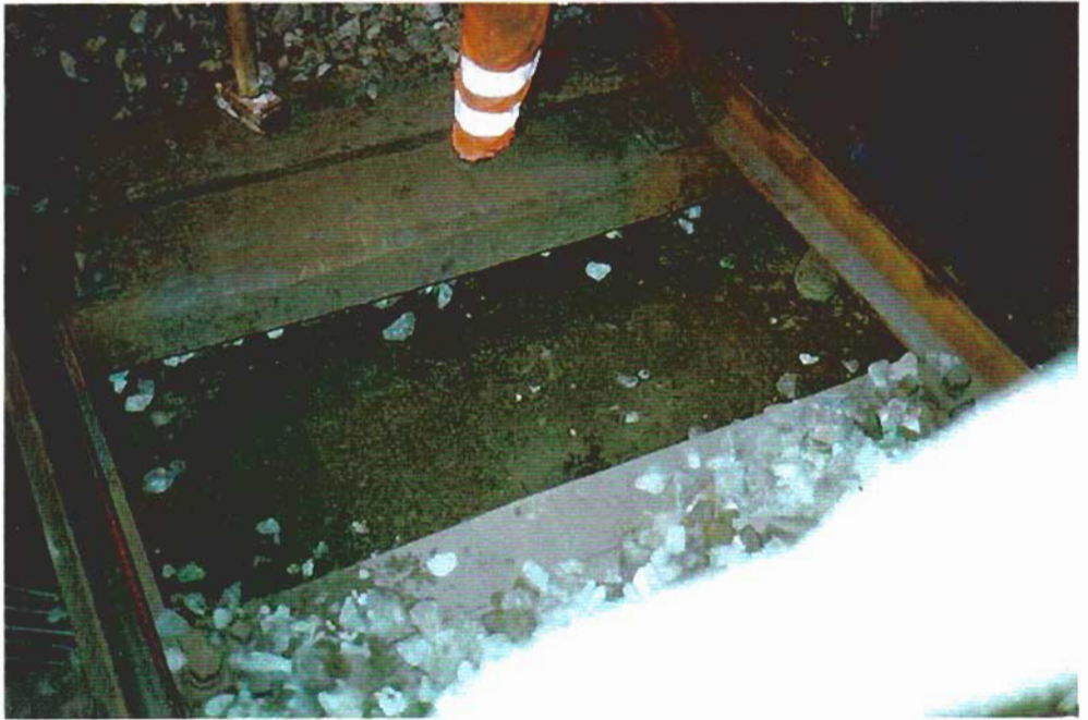
Fig. 1: Removing of the SBM - opening of the sleeper spaces
