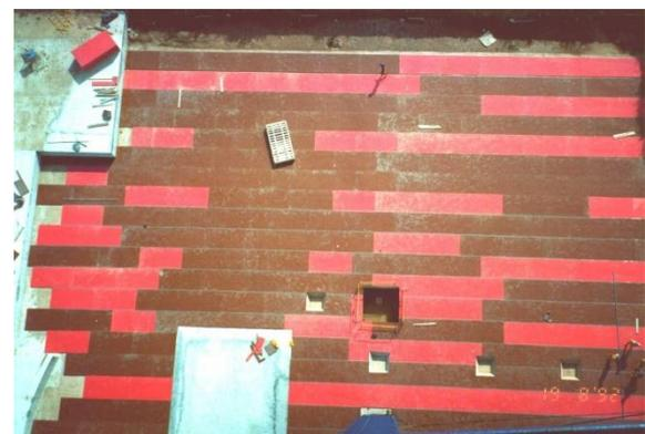
Fig. 3: Installation of Sylomer® 1991/92
