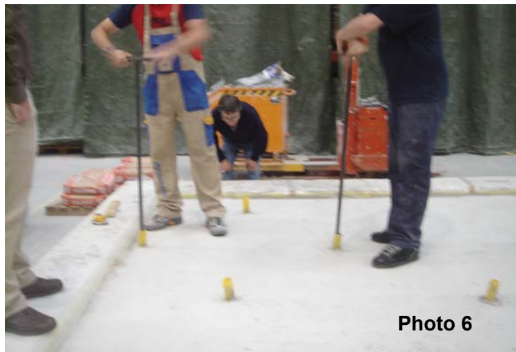
Photo 6: Raising of concrete slab
