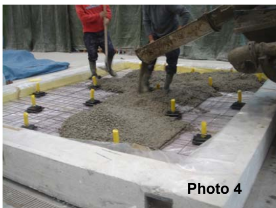
Photos 4 and 5: Spill of concrete
