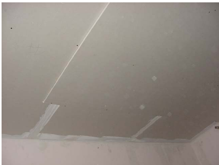
Photo 4: Mounting of the third plasterboard
