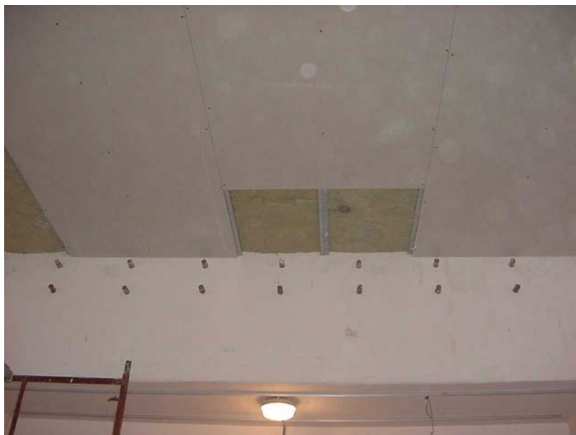
Photo 4: Mounting of the first plasterboard
