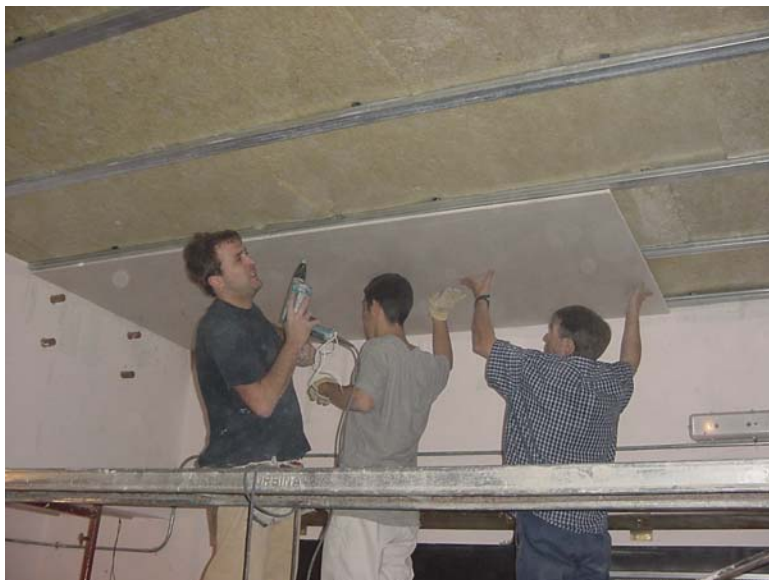
Photo 3 : Mounting of plasterboard
