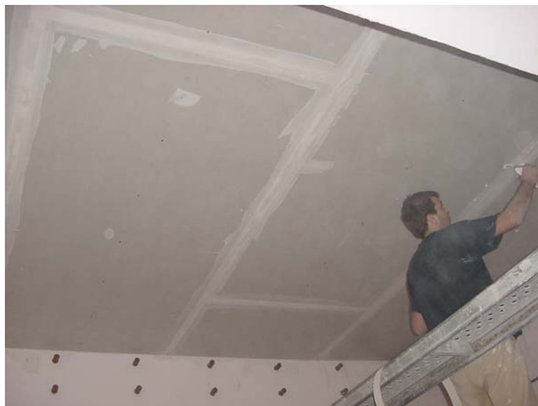
Photo 4 : Sealed of joints
