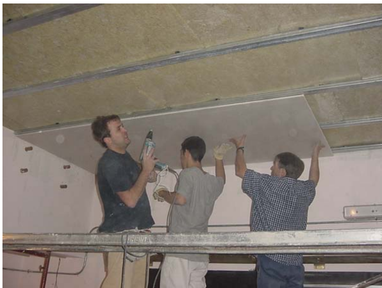
Photo 3: Mounting of plasterboard
