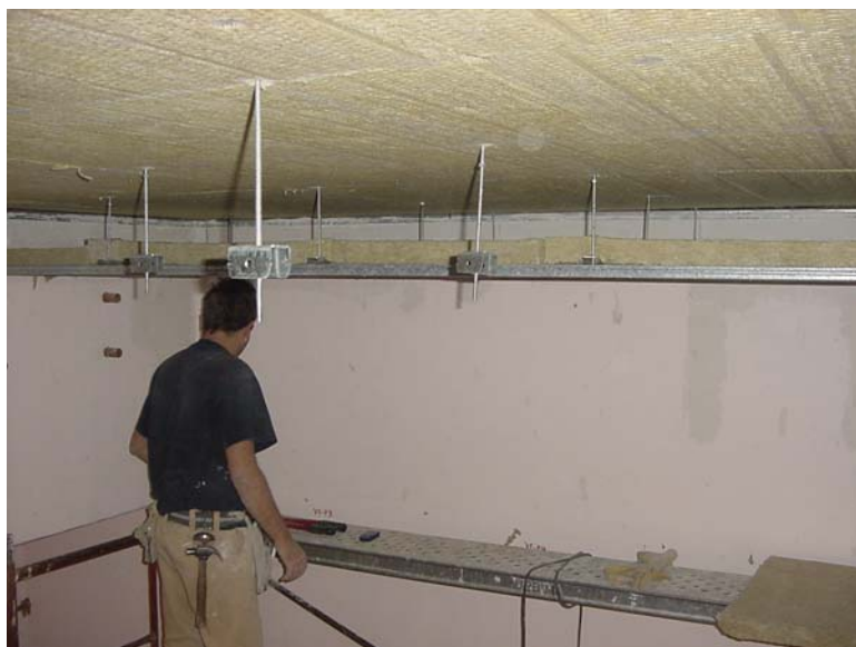
Photo 2: Mounting of rods, profiles and second layer of rock wool
