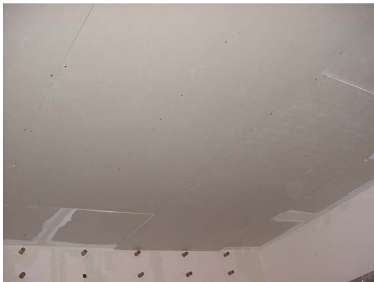
Photo 4: Mounting of the third layer of plasterboard
