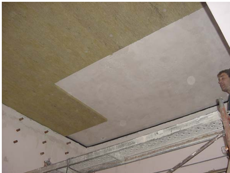
Photo 1: Mounting of the first layer of rock wool
