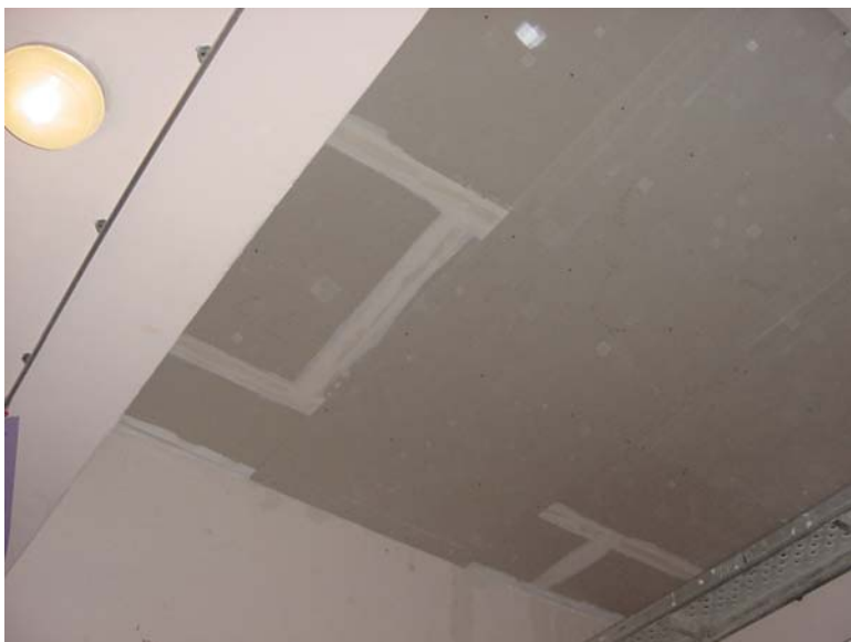
Photo 4: Mounting of the second layer of plasterboard
