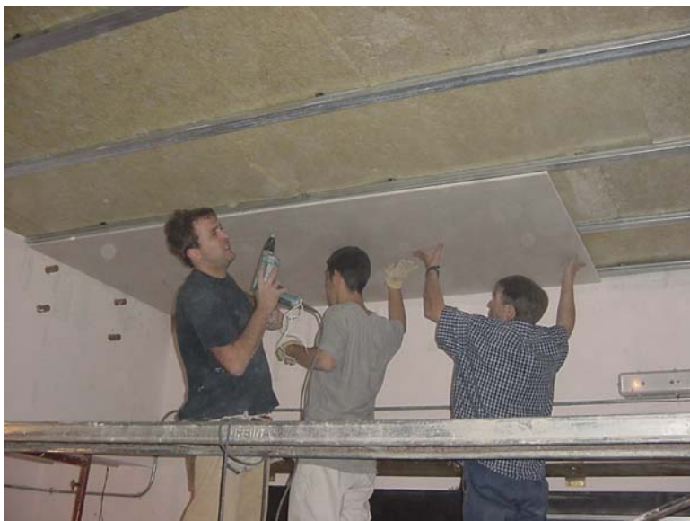
Photo 3: Mounting of plasterboard
